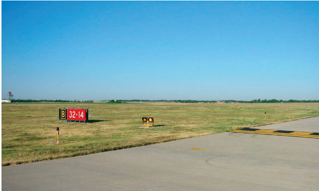
Holding position for Runway 14-32 on Taxiway Bravo. An above ground runway guard light is installed between the holding position sign and pavement marking.
