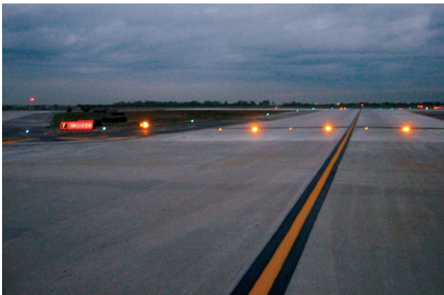
Runway holding position as viewed from a taxiway centerline. This holding position has both above ground and in-pavement runway guard lights.
